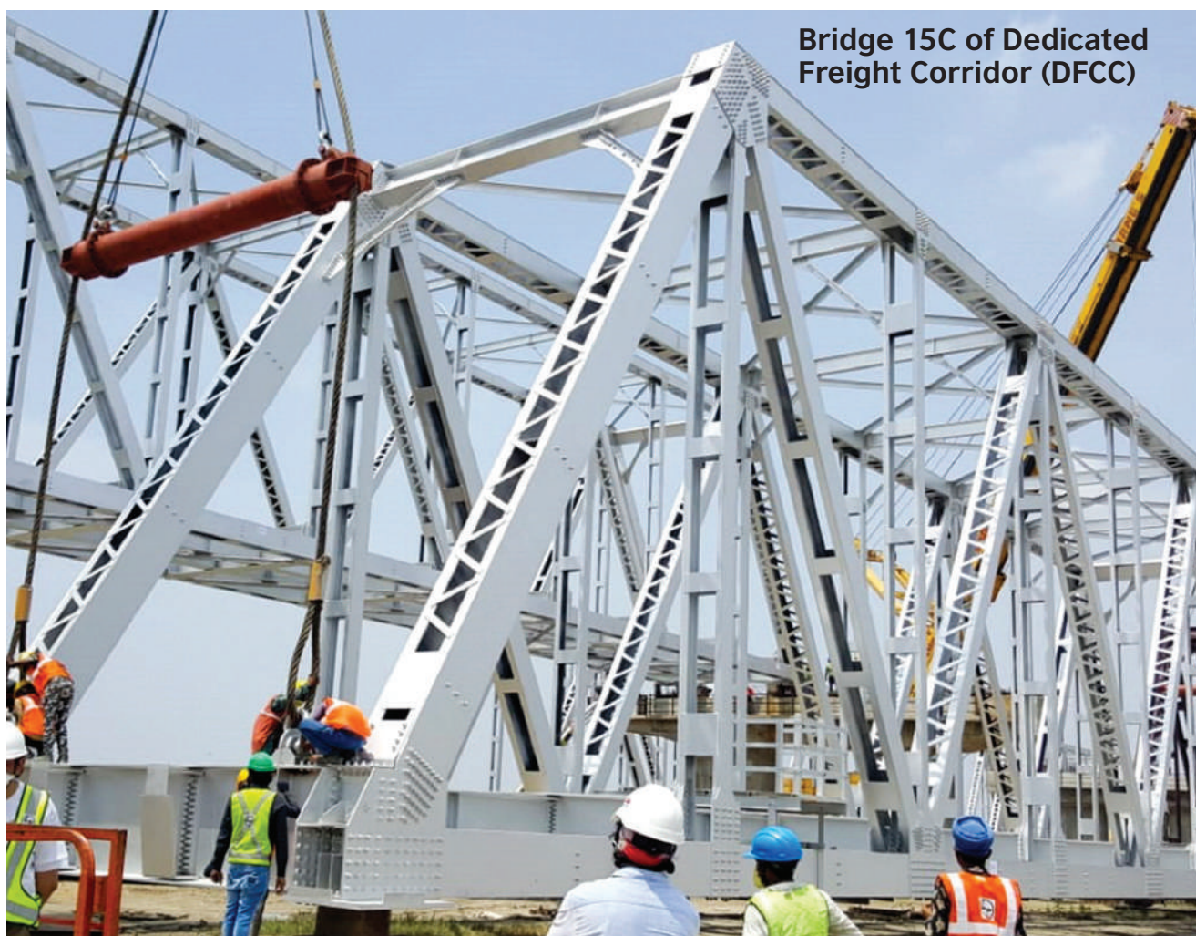
Launching of Twin Box Open Web Girder, 441 MT, Mumbai
